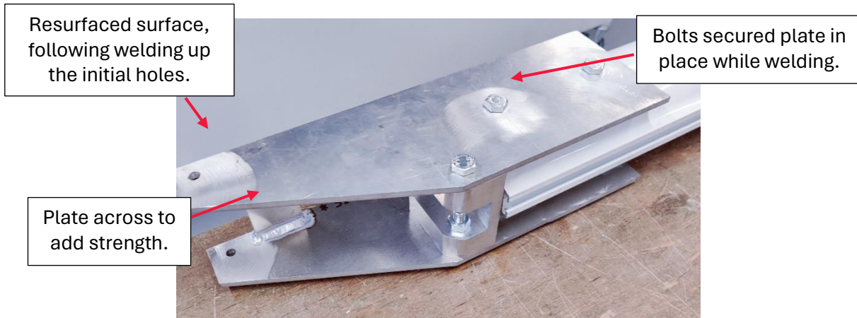
Figure 65 - Side plates secured in place.
